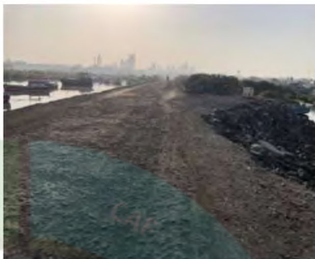
Approach Road for Literage Jetty.
