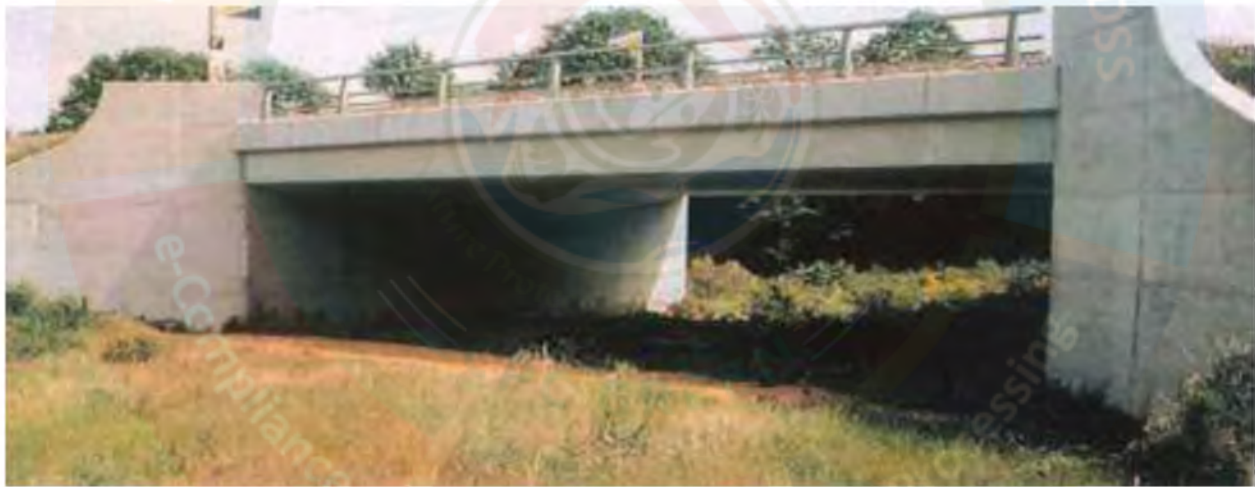
Figure 7: Example of an underpass below highway with good openness index and suitable for the movement of large mammals as well as other wildlife species of the landscape. (Google images).
