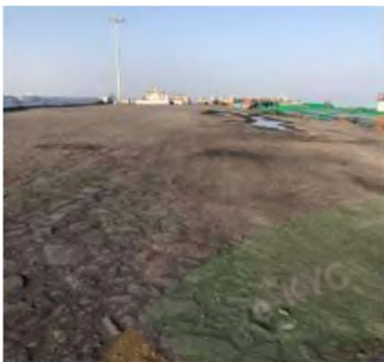
Existing Literage Jetty.
